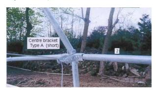
Assemble the frame on the ground as before, no compression tube brackets should be fitted.
