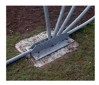
Assemble the frame on the ground as before, bearing in mind that the Compression tube brackets should be fitted to the centre bracket so there will be one central 1544 mm Compression tube going to frame 5 and one to frame 3.
