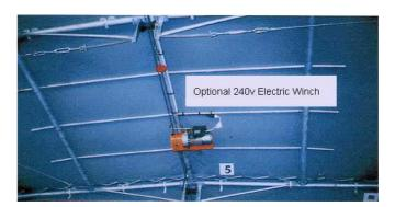
These are simpler frames without the tension reinforcements, the same as frames 3, 2 & 1 except they all have 2 winch rollers. Assemble the frame on the ground as before, bearing in mind that the top brackets should be the same orientation as you fitted on frames 6 & 7 so the chain is always on the same side.
